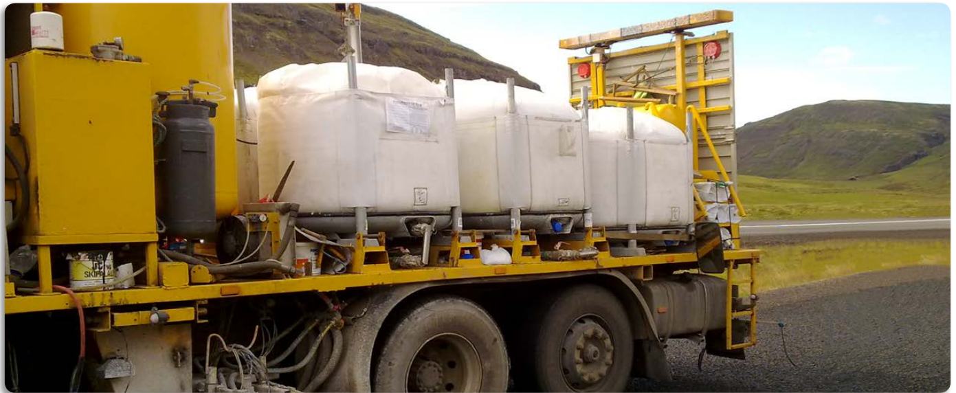
Fluid-Bag Multi containers on paint truck
