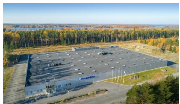
Fluid-Bag Ltd headquarters and main production facility.
