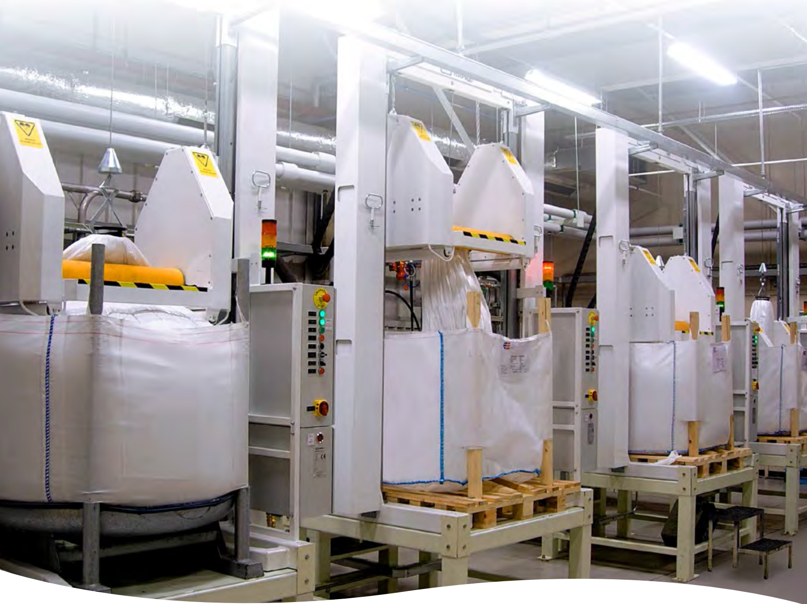
Toyota's manufacturing plant in Burnastone UK where Fluid-Bags are used for sound damping pastes for vehicles. Automated Fluid-Bag Discharge Rollers empty the bags and are connected directly to the vehicle production line.
